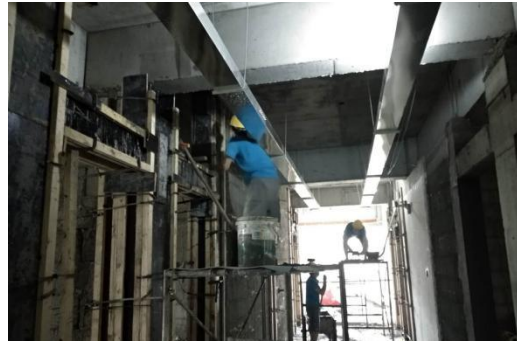
构造柱浇筑
