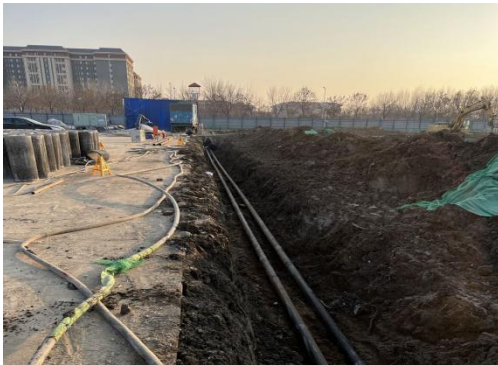
场地周边管线敷设
