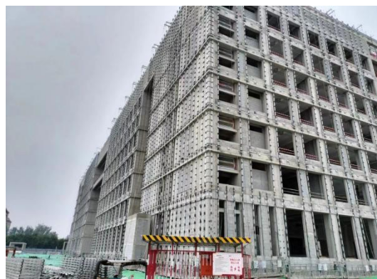
幕墙龙骨安装
