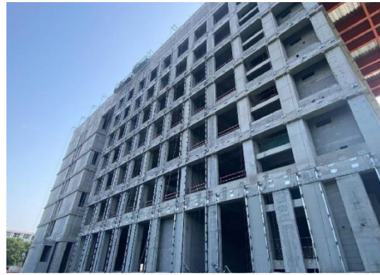
幕墙龙骨安装
