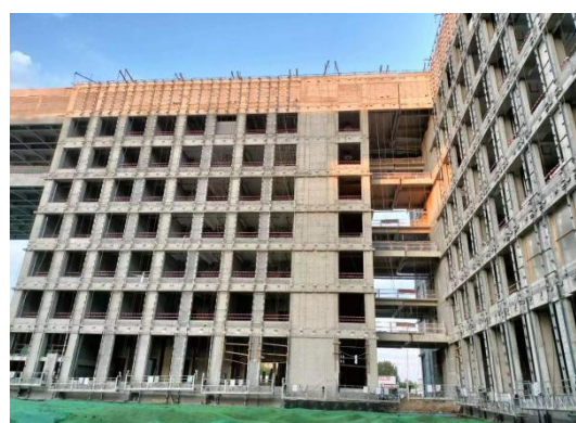
幕墙龙骨安装
